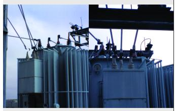
Thermal imaging technology can make it easier to assess the health of an LTC by quickly revealing hot spots
