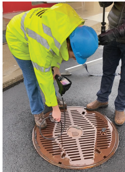
Figure 8.1 Inserting the probe into the test area.
