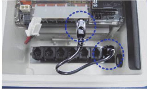
Installing Connector Cable
