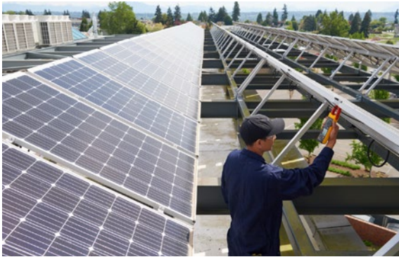
The Fluke 393 FC can measure voltage, current, dc power and provide audio indicator for incorrect polarity on PV panels.
