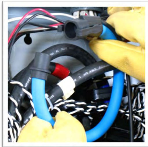
Photo 2: Install CT Around Conductor.
