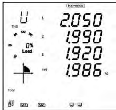
Figure 3-21 - Harmonic Distortion Reading
