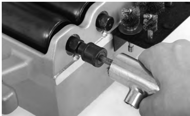
Figure 14 – Cleaning Inside of Fittings
