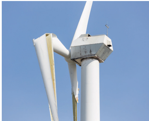
Figures 2a and 2b: Damage from lightning strikes on wind turbines
