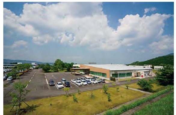
Figure 49 Mitutoyo Miyazaki Plant, Co., Ltd.
