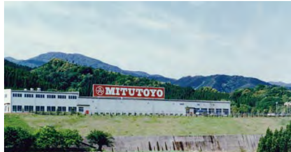
Figure 37 Miyazaki Mitutoyo Precision Co., Ltd. (presently Mitutoyo Miyazaki Plant Co., Ltd.)
